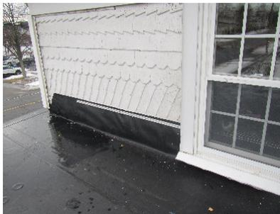
The contractor did not properly fasten the roofing perimeter that contacted the exterior walls of the second-floor of the home.
